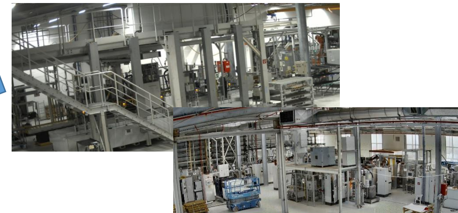
View on the Module production line
